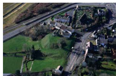
Aerial view of Loughor Castle & Town © Crown: RCAHMW
