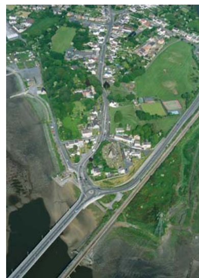
Aerial view of Loughor © Crown: RCAHMW
